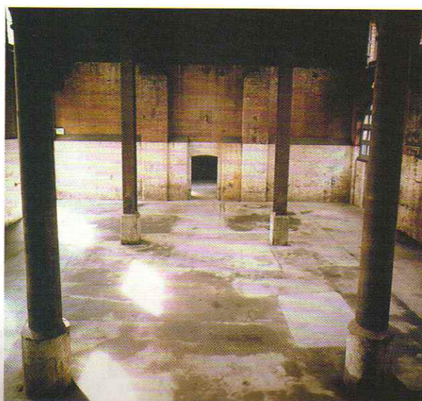
Wapping Hydraulic Power Station pre-installation
